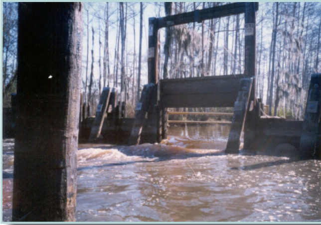
A sluice gate alleviates flooding and allows freshwater to be introduced into stressed swamps.
