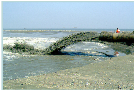
A dredge discharges sediment onto Wine Island.
