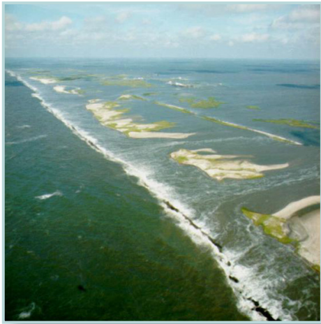
Overwash and breaching of East Timbalier Island, showing limited effectiveness of the breakwater during extreme storm events.
